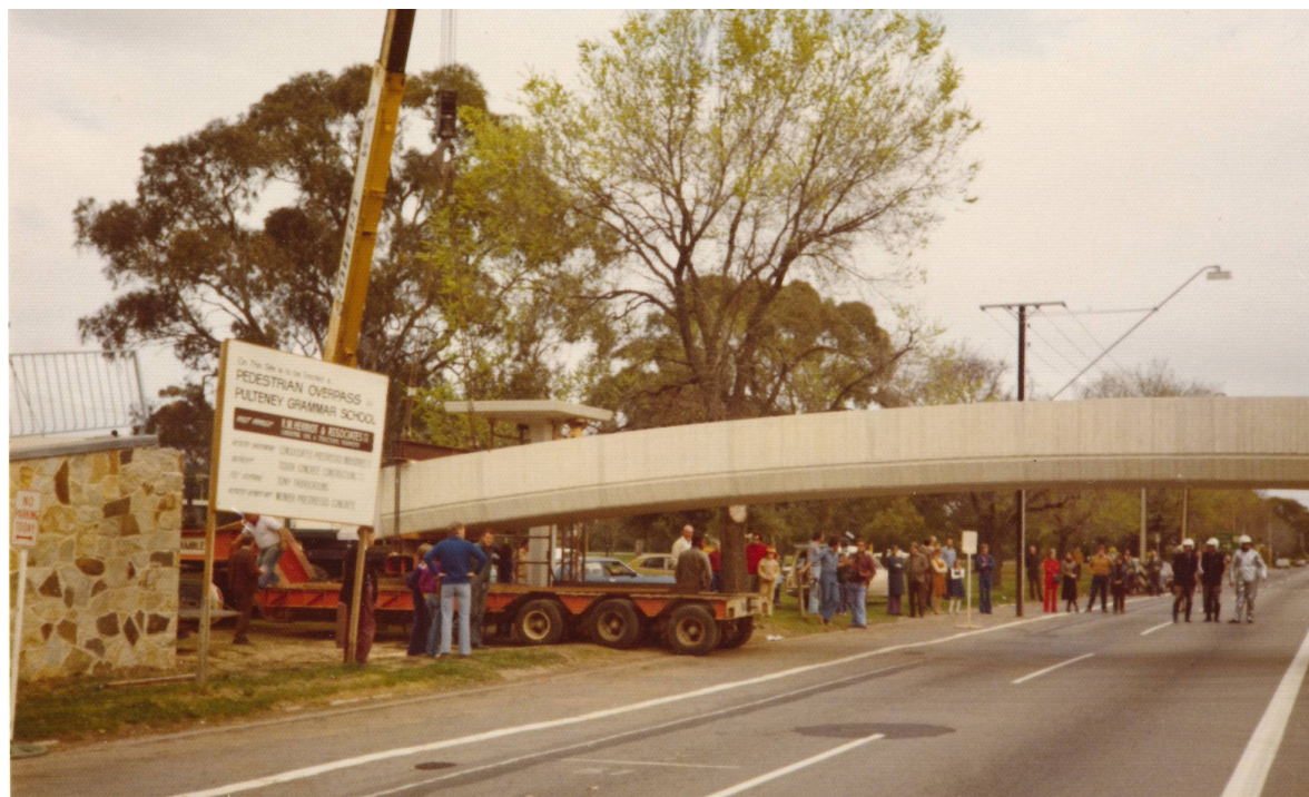
Lifting the overpass into position, 19 September, 1976.
